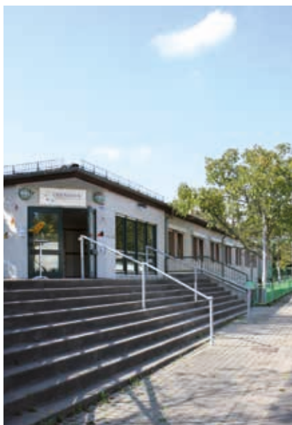
International School – Campus Frankfurt
