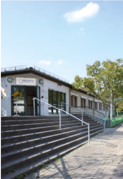
International School – Campus Frankfurt
